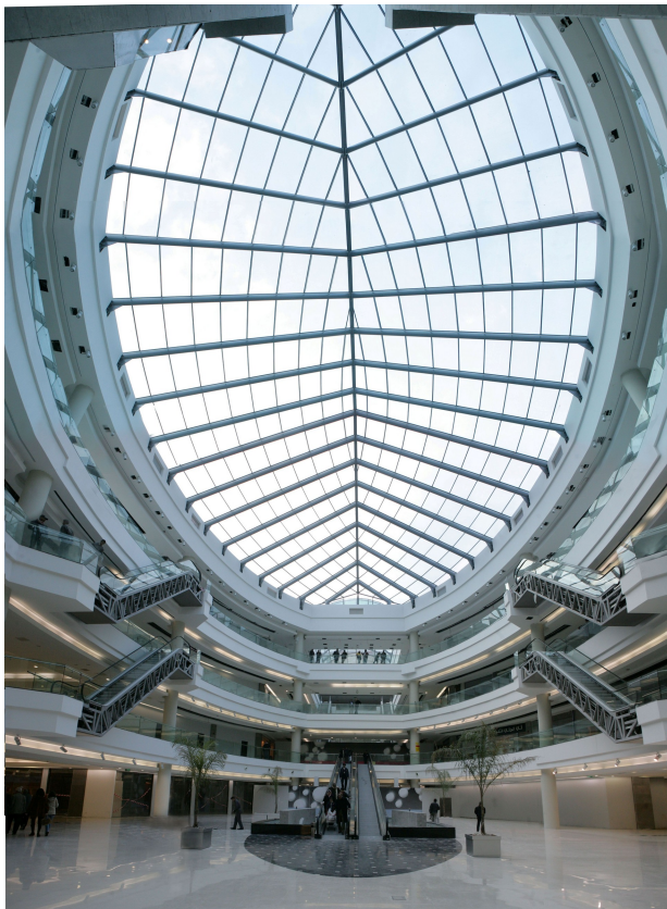
Skylight City Mall
